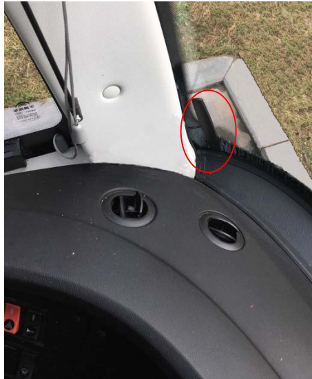
Figure 2-16 Inside installation of Mobile Network Antenna
