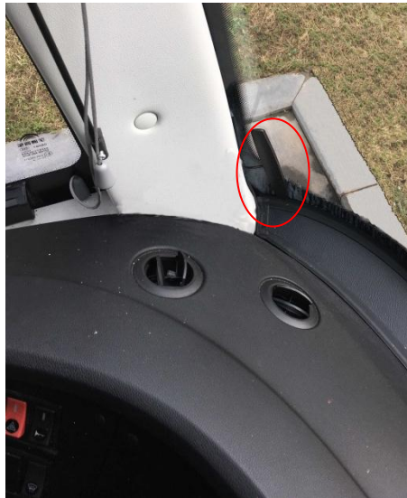
Figure 2-17 Inside installation of Mobile Network Antenna
